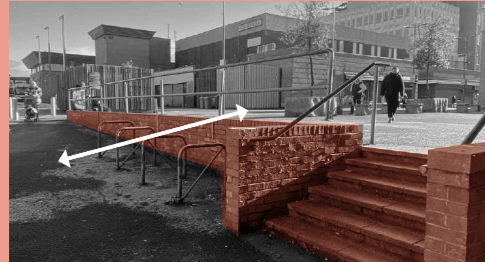
Level change poorly addressed, pedestrians channelled down steps creating a disconnect with Queen's Walk
