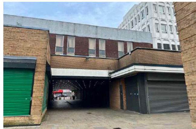
Voids within the buildings
